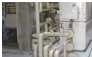
Bathroom heating system with filtration unit
