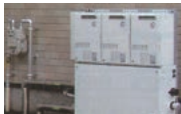
■ Hot water circulation system
