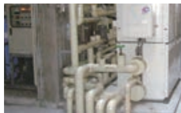
■ Bathroom heating system with filtration unit
