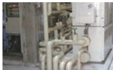
Bathroom heating system with filtration unit
