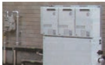
Hot water circulation system
