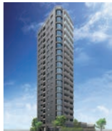
XESTA TOWER NAGOYA DAIKANCHO
