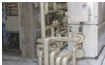
■ Bathroom heating system with filtration unit
